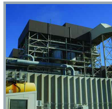
The recently acquired Twin Oaks power plant provides Sempra Energy Resources with fuel diversity and entry into the Texas power market.
