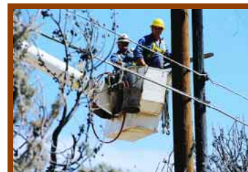
In August 2002, SDG&E workers battled difficult conditions to replace power poles and other equipment damaged in a fire that burned more than 60,000 acres in eastern San Diego County.
