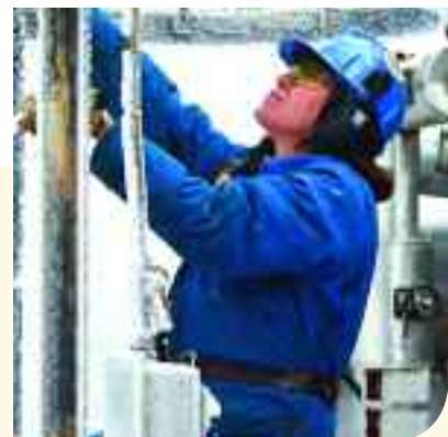
From left to right: Employees performing a leak-detection assessment; monitoring a control panel at Cold Lake; working safely at the Nanticoke refinery.
