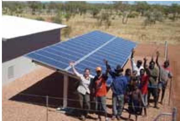
Solar panel installation at a Bushlight community, Northern Territory, Australia
