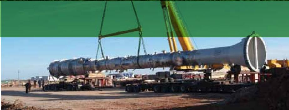
A demethanizer tower is installed at Devon's 200 million cubic feet per day gas processing plant in the Cana-Woodford Shale. By owning and operating gas processing facilities, Devon can improve its operating efficiency.
